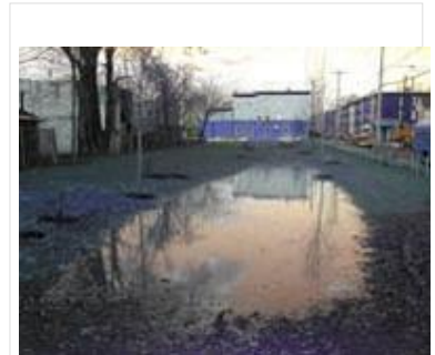
This vacant lot in Philadelphia was regraded to direct runoff into strategically placed swales and depressions. (Photo courtesy of Philadelphia Water Department)
